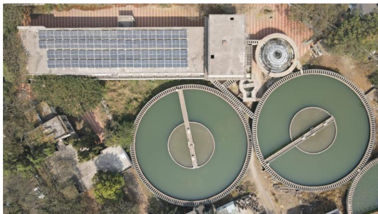
Figure 11-1 Installation of Rooftop Solar System at WTP
