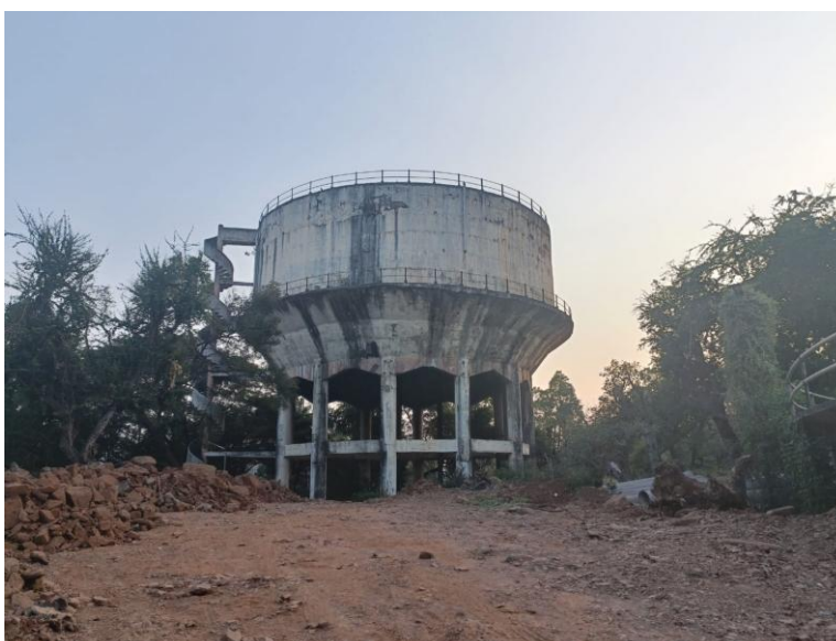
Figure 4-3 Elevated Service Reservoirs at Ichalkaranji City
