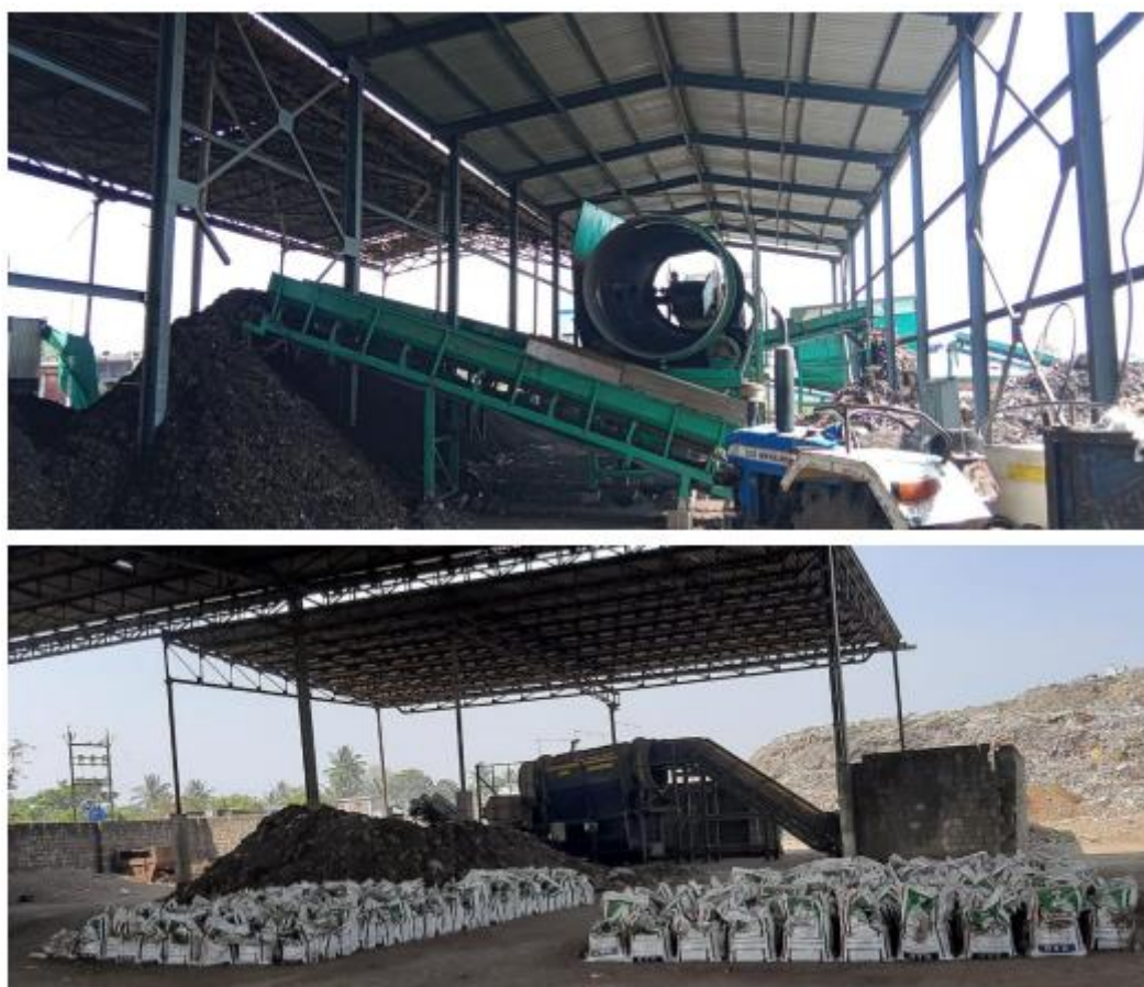
Figure 9-3 Wet Waste Processing Unit
