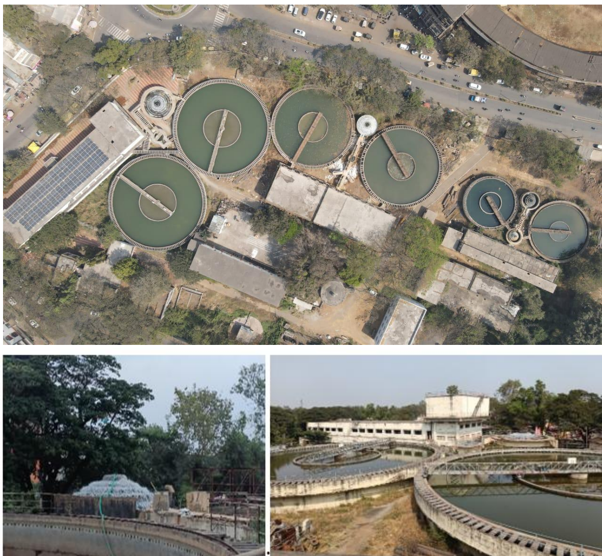
Figure 4-2 Photographs of Water Treatment Plant at IMC
